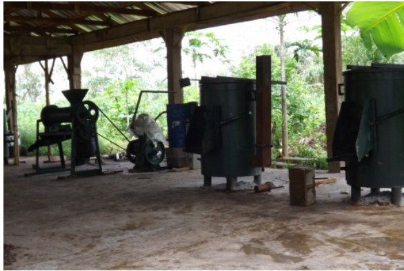
Figure 4: The NIFOR processing equipment is installed in the new mill building.
