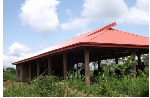
Figure 3: The newly completed mill building just after completion in May 2012.
